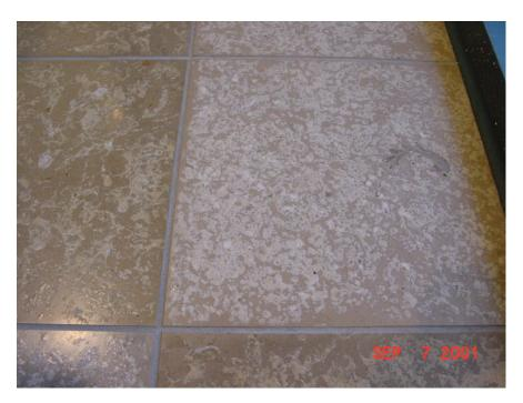
PROCON utilizes moisture vapor detection devices to detect and avoid costly failures of moisture sensitive finishes such as the limestone tile shown above
