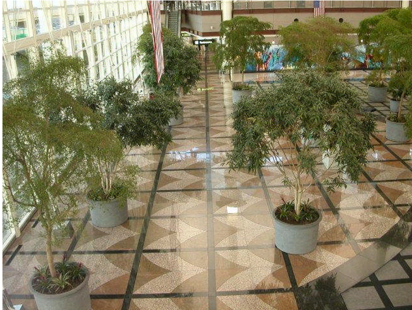
Figure 4 – polished finish granite is durable in high-traffic airport retail area, but even hard, dense stones will eventually show wear
